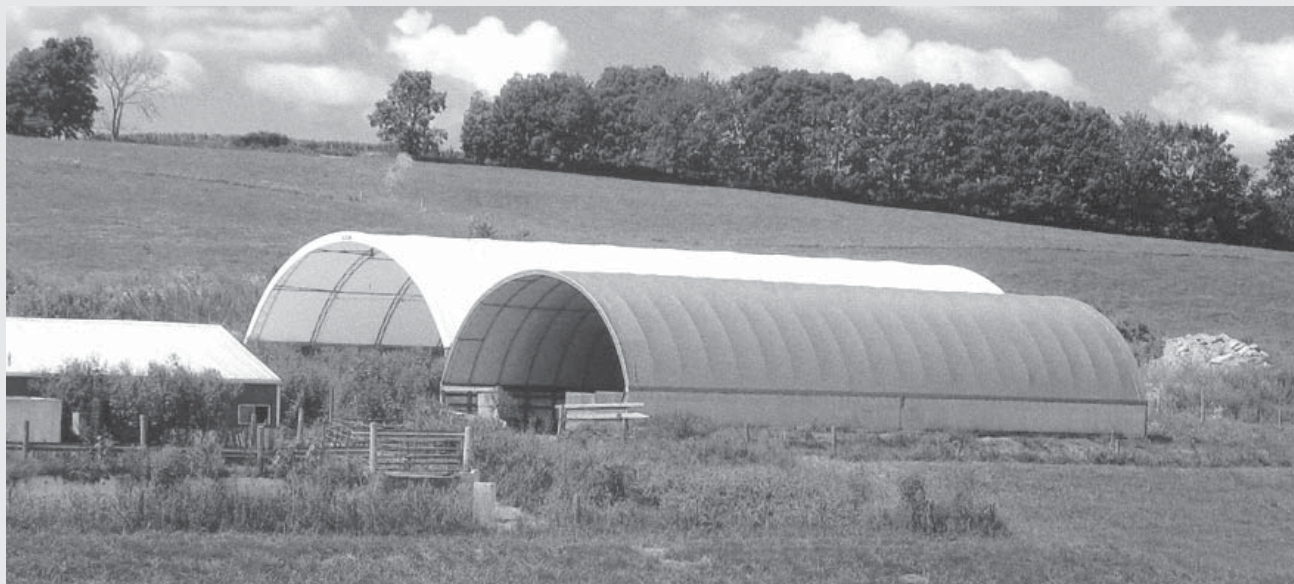
The Vosbergs constructed two canvas hoop sheds to provide shelter on bedded packs during the worst winter weather.
