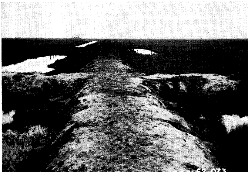
FIGURE 3. Earthen levees with staggered borrow pits improve accessibility of marsh range and enable cattle to graze range evenly.
